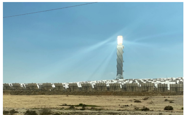
The Ashlim solar power station in the Negev desert
